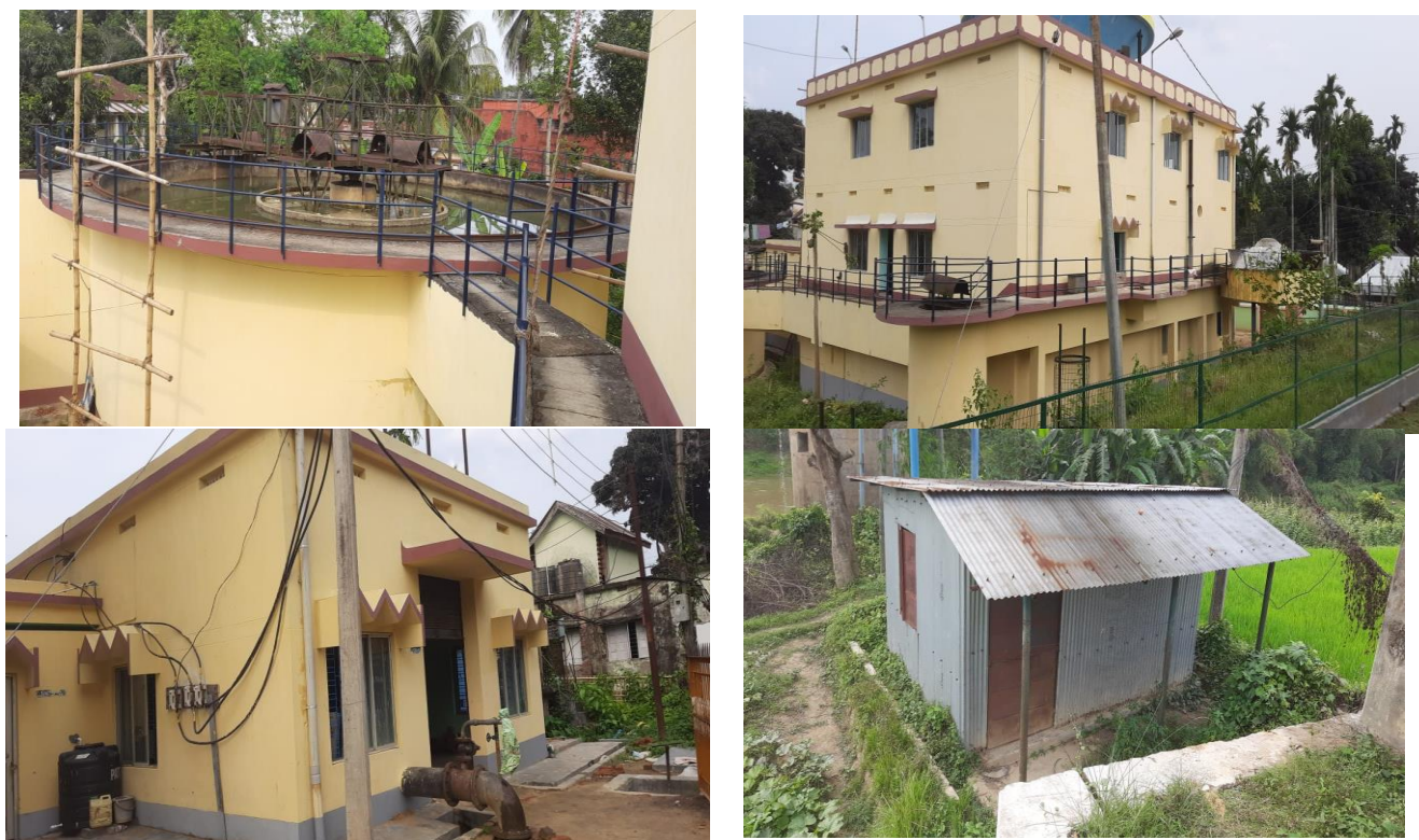
Photograph of Intake at Amarpur
