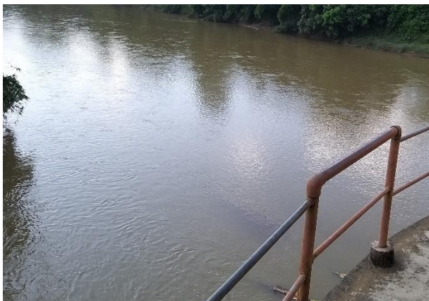
Existing Intake on River Gomati
