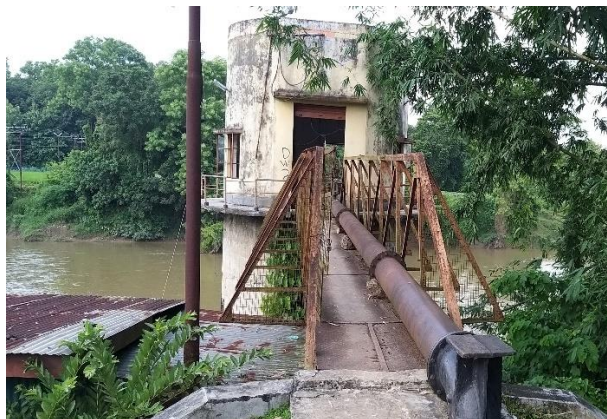
Existing Intake on River Gomati
